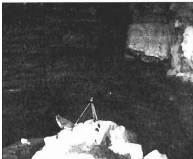
Fig. 8 - St Michael's Cave, looking west. The dyke is the vertical dark band in the background just right of centre. The tripod is on top of a fresh breakdown cone produced by major ceiling failure along the dyke in 1980. Blocks in the pile are sandstone, the clastic dyke material weathers to form black silty sand. Note failure along horizontal bedding planes in the upper right of the image.
